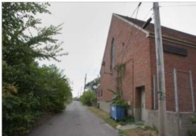
Workers will repave this alley that runs parallel to University Avenue between St. Albans and Dale streets in St. Paul with money from the Central Corridor project's contingency fund. (Staff photo: Bill Klotz)
