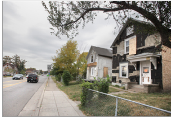
The Bottineau transit route known as D2C would require 110 or more homes and businesses to be demolished on the west side of Penn Avenue between West Broadway and Olson Memorial Highway to make way for light rail transit trains on Penn Avenue — like these. (Staff photo: Bill Klotz)
