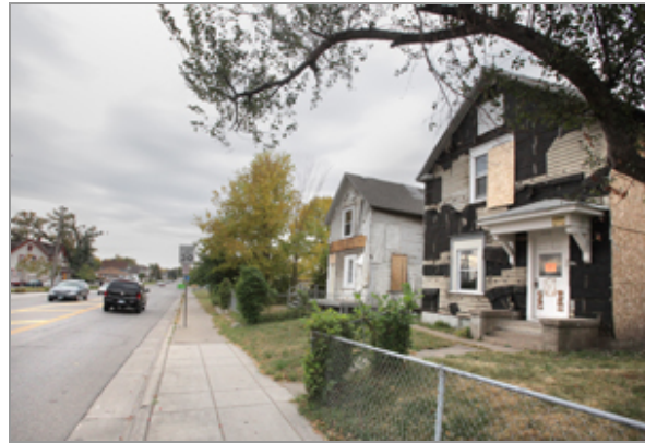
The Bottineau transit route known as D2C would require 110 or more homes and businesses to be demolished on the west side of Penn Avenue between West Broadway and Olson Memorial Highway to make way for light rail transit trains on Penn Avenue — like these. (Staff photo: Bill Klotz)
